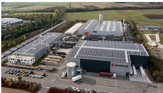
At the Knetzgau site, the PV systems are clearly visible.
