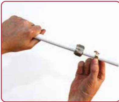
4. Place the nut and olive onto the pipe.
