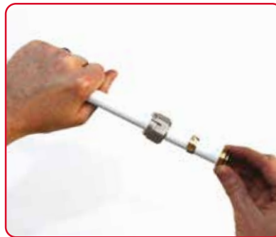
5. Push the fitting into the bevelled end of the pipe.
