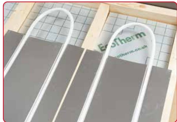
2. Roll-out the pipe into the required pattern and fit into the Heat emission plates.
