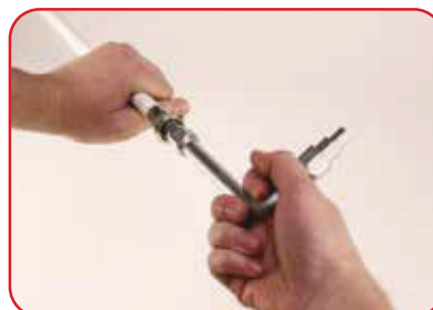
5. Use the allen key to screw the thread into the pipe.
