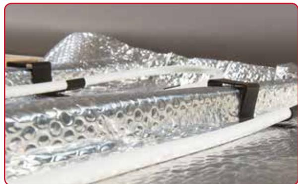
2. Roll-out the MLCP pipe into the required pattern and secure on the Mainfoil clips.
