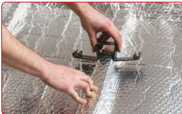
1. Fit the Mainfoil to the top of the joists and secure with Mainfoil clips at 200mm centres.
