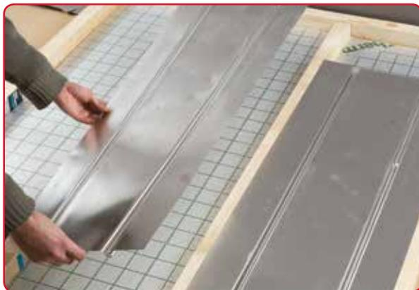
1. Heat emission plates laid between the joists at 400mm centres and secured using suitable fixings.
