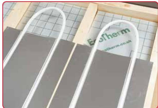
2. Roll-out the pipe into the required pattern and fit into the Heat emission plates.
