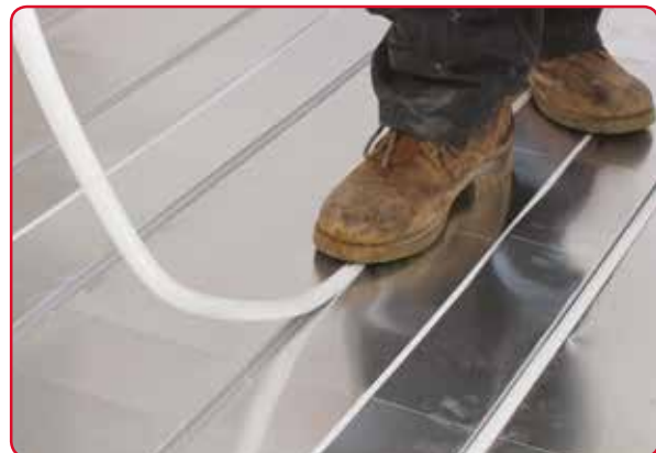
2. Roll-out the pipe into the required pattern.
