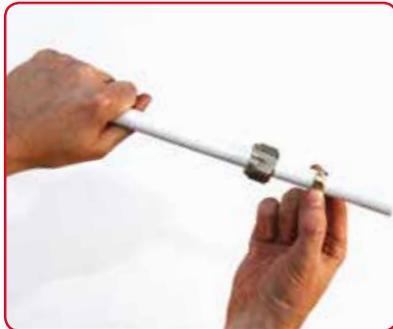
4. Place the nut and olive onto the pipe.
