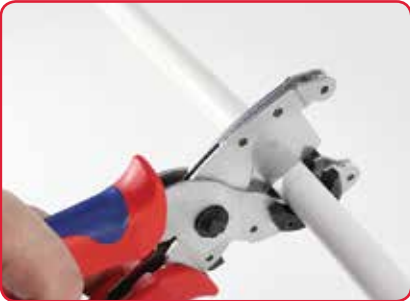
1. Cut the pipe at a 90° angle
